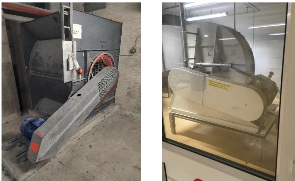
Figure 8 Example of belt-driven ventilators.
