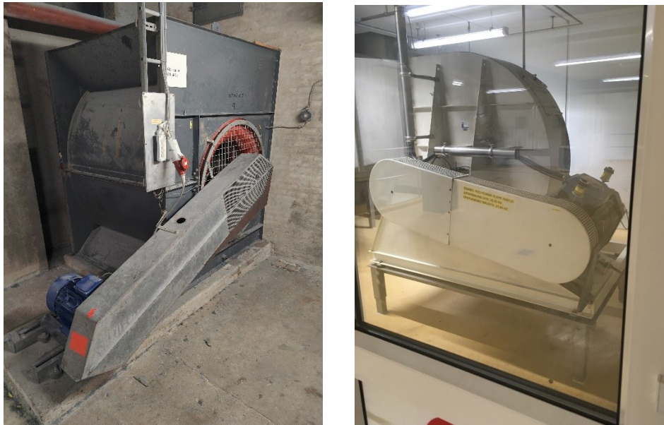
Figure 8 Example of belt-driven ventilators.
