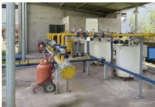
Figure IV.16. Electric LPG vaporizer
