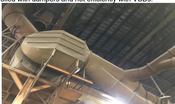
Figure 3-10: Large exhaust fan in an iron & steel industry
