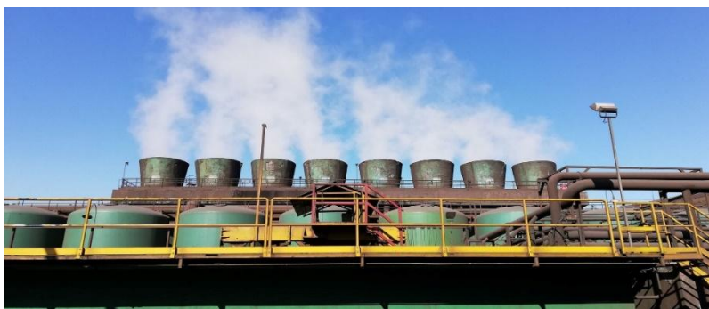
Figure 3-12: Cooling water system in an iron & steel industry
