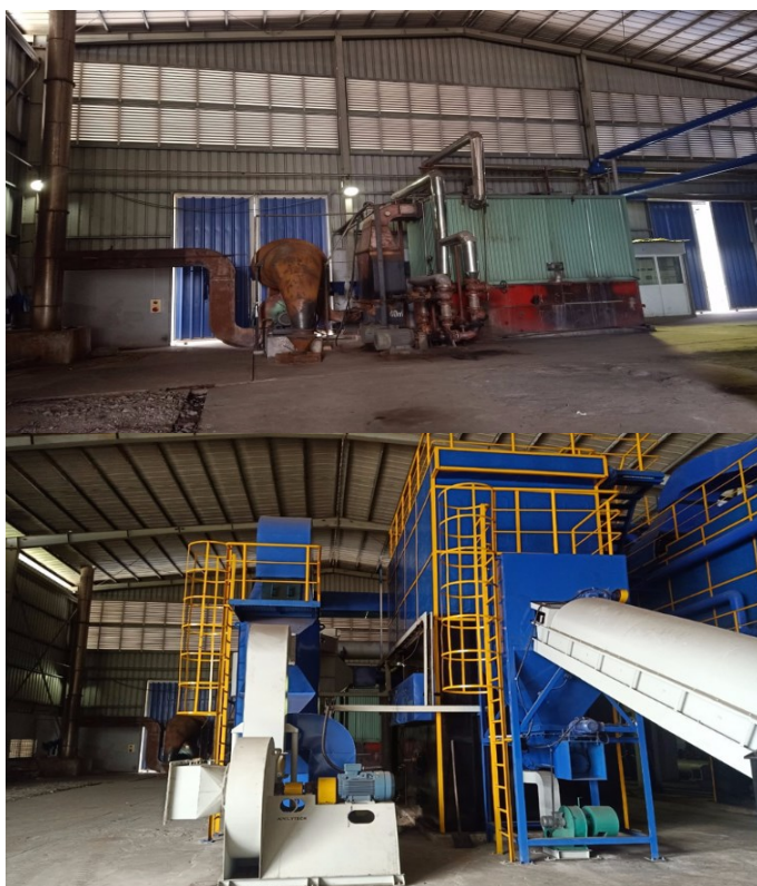
Figure 9. New high-efficiency hybrid boiler for use of biomass (and coal)
