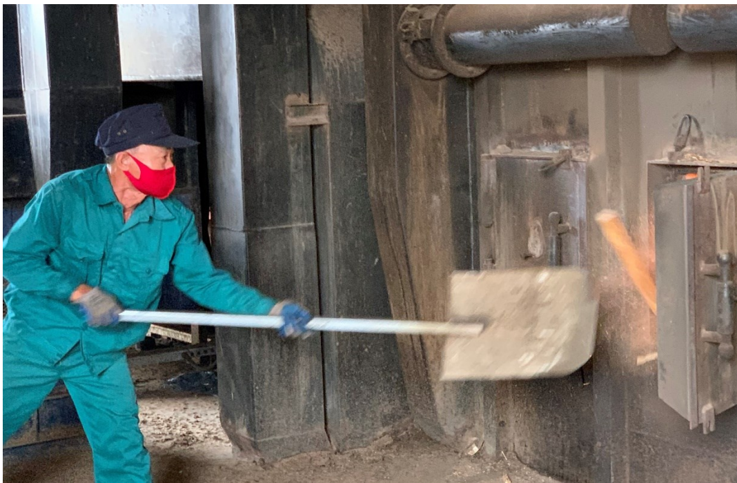
Figure 1 Example of manually fed boiler
