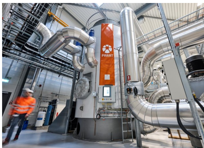
Figure 13. Example of an electro boiler installation.
