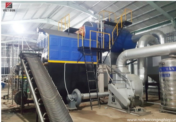
Figure 11. New wood pellet boiler to replace oil boiler
