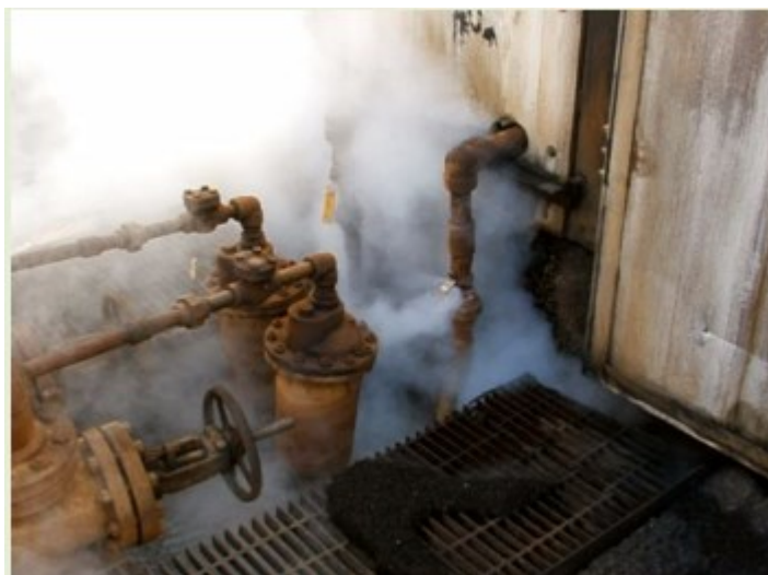
Figure 7. Example of leaks from a steam distribution system
